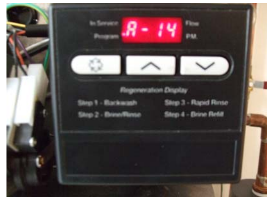
Fig 4 If 2000 gallon backwash isn't reached in certain amount of time, the system will backwash after set amount of days (14 days in Fig 4) regardless of remaining water.
