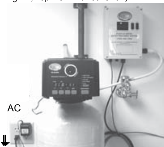
Figure 1B. Your ECOsmarte® Software Version. Enable the valve by connecting the wall AC-adaptor to the water valve at the lower left, your software version will display. (Fig. 1B, Above) Depress the set button to go to step 3. (Fig.1C, Below)
