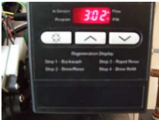
Fig 1 Time and Day. Ecosmarte® Control Valve is displaying the time of day.
