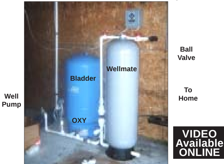
Fig. 2: Oxy Chamber Plumbed Prior to Wellmate or Dynamixer In All Installations.
