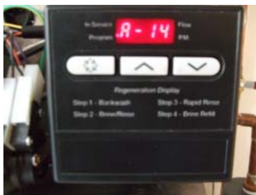
Fig 4 If 2000 gallon backwash isn't reached in certain amount of time, the system will backwash after set amount of days (14 days in Fig 4) regardless of remaining water.
