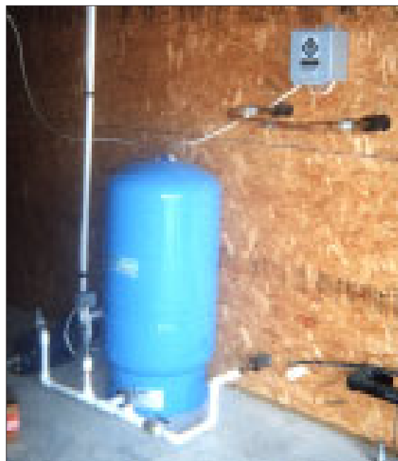
Fig. 1: Free Space to allow for proper backwashing; Anchor 1/2" drain hose from water valve to drain. Water must backwash at 10 gpm. Backpressure from undersized drains must be avoided (well pump to bladder tank shown above, pre-install).
