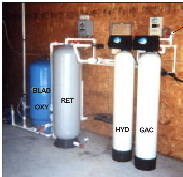
Fig. 3: Left to Right: Wellmate, Well, Bladder Tank, OXY Chamber, Hydroxite Tank, Carbon Tank, Flow Switch, Cu Chamber (behind GAC), Water to Home.
