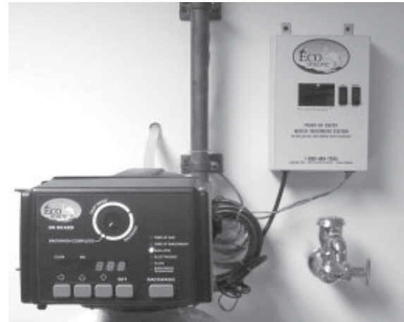
Figure 4. Remaining gallons to backwash. Ecosmarte® Control Valve is displaying the remaining gallons to backwash, as indicated by the green LED on the right. The green LED for gallons will remain constantly lit when the programmed filter life has been entered in years (7) or in gallons (500,000). ver. 1.2, Sept-2003)
