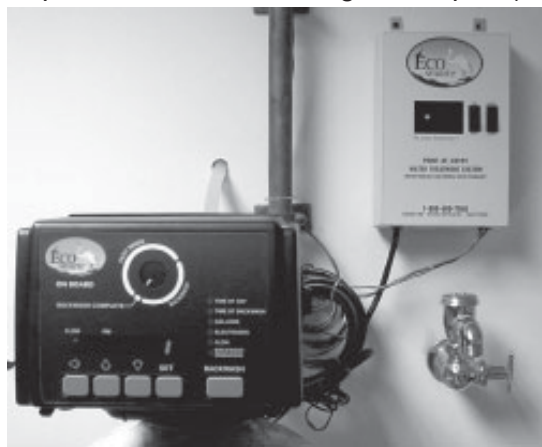
Figure 1C. Setting Time of Day and Choosing Time of Backwash. Working right to left on the display, the up and down arrow keys allow you to set the column value. Press the left arrow to move to the next column. When all columns are finished, press the SET key.
