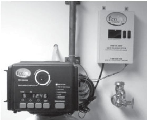
Figure 2A. Time and Day. Ecosmarte® Control Valve is displaying the time of day AND the day of the week. (5=Thursday)
