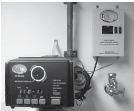
Figure 1B. Your ECOsmarte® Software Version. The version of your software is displayed. As updates, upgrades, OR regulatory changes occur a simple board changeout at nominal charge will keep you in the latest technology. Depress the set button to go to step 3. (Fig.1C, Below)
