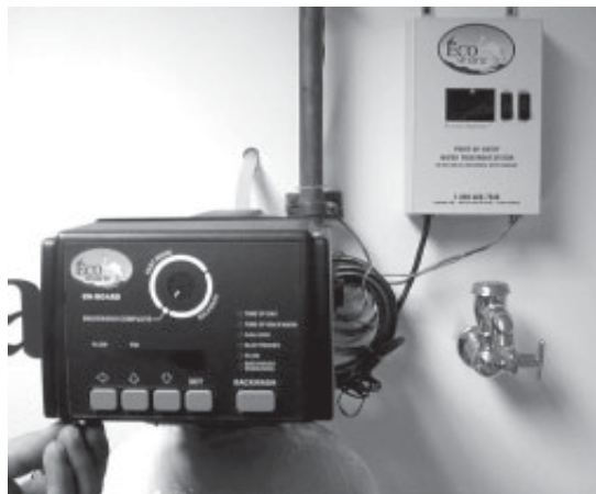
Figure 1A. Activating Your ECOsmarte® Control Valve. Enable the valve by connecting the wall AC-adaptor to the water valve at the lower left, your software version will display. (Fig. 1B, Below)
