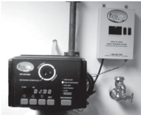
Figure 1D. Ecosmarte® Control Valve is displaying the time set for backwash (02.00AM). Backwash starts automatically when the preset usage has been reached, at 2.00AM when total gallons have been used that day.
