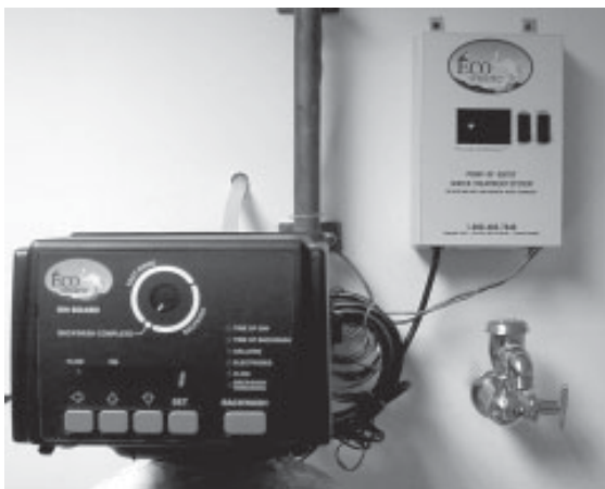
Figure 2B. Household Water Demand. Ecosmarte® Control Valve is displaying the total flow rate (1 GPM) demanded by the property in gallons per minute. The ECOsmarte® control box lights circle (above right) when ever water is demanded above ½ GPM. A one to four second delay occurs.
